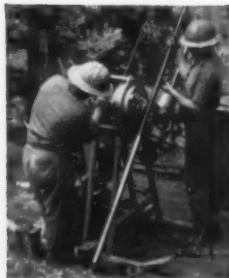
Full 360° swivel head permits drilling at any angle. The hinged drill head swings out of the way and the powerful drum hoist conveniently lifts or lowers drill rods when adding or removing drill rods.
